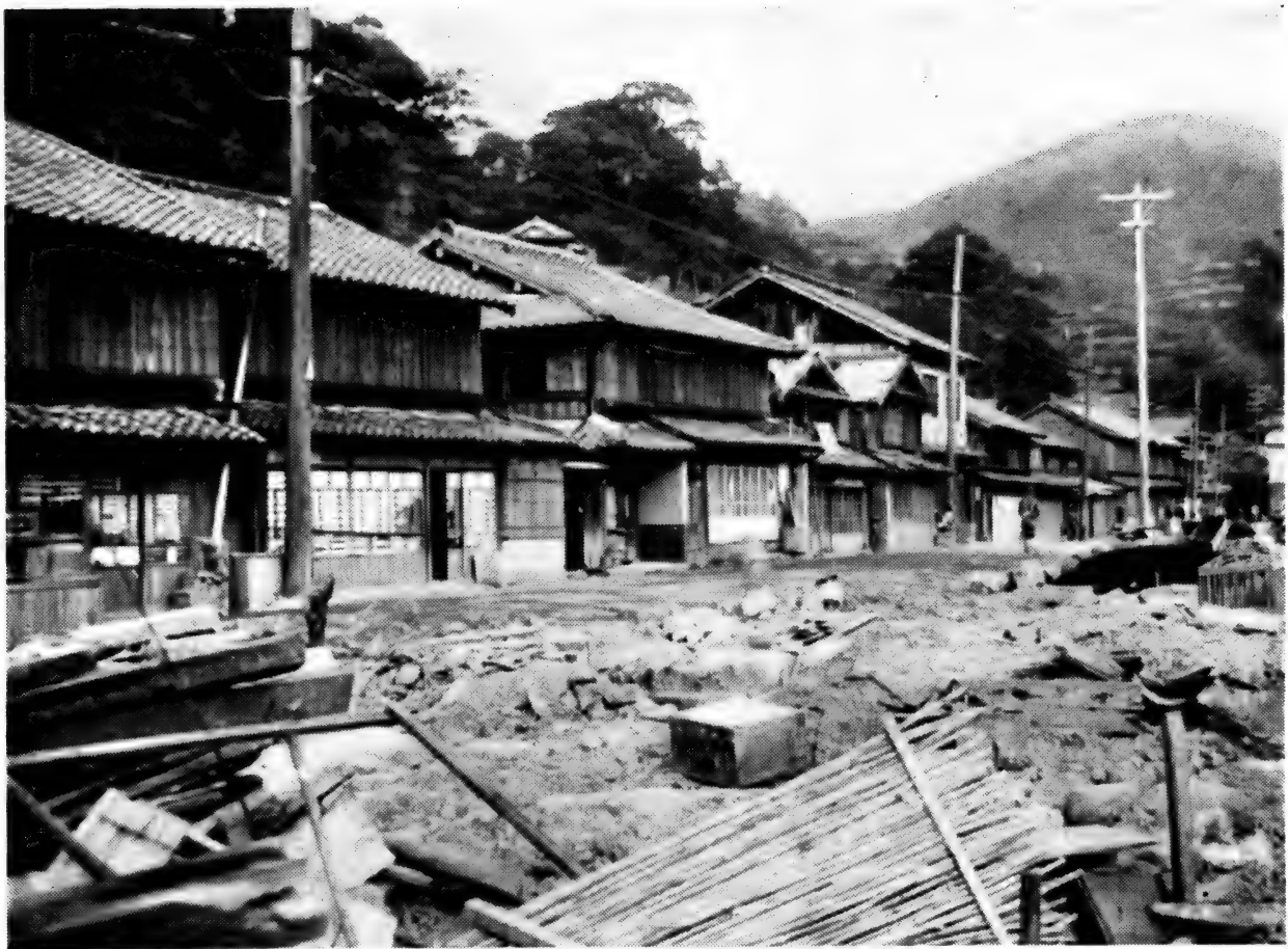
Photo No. 19. NAGASAKI. Typical Japanese houses in a street screened from damage by the surrounding hills. Buildings of similar construction formed the main proportion of buildings in Nagasaki and Hiroshima. See paragraphs 37 and 80.
